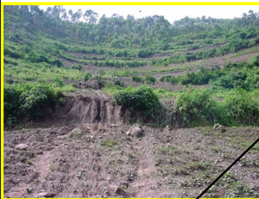
Severe run off
